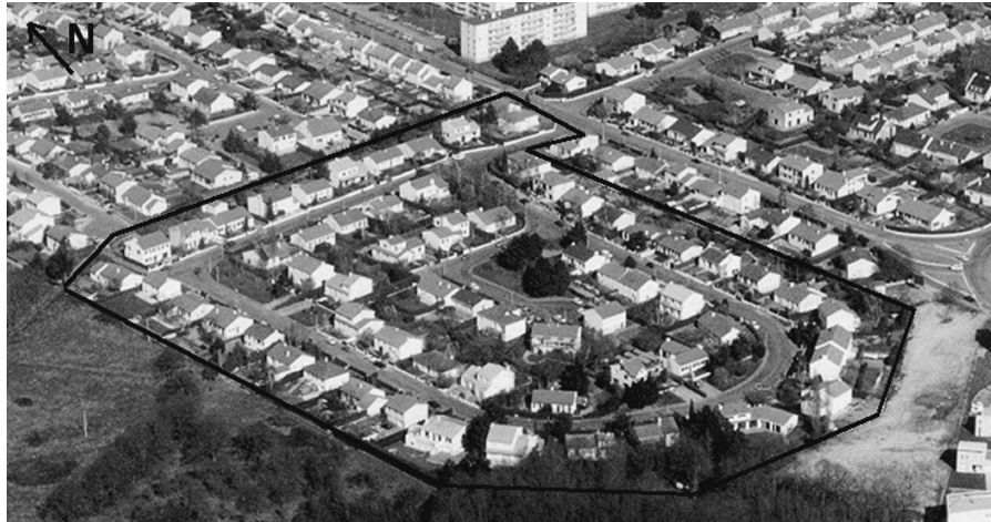
FIG. 2. Aerial view of the Rezé site. The black continuous line indicates the limits of the catchment drained by the drainage network in the right-hand corner.
